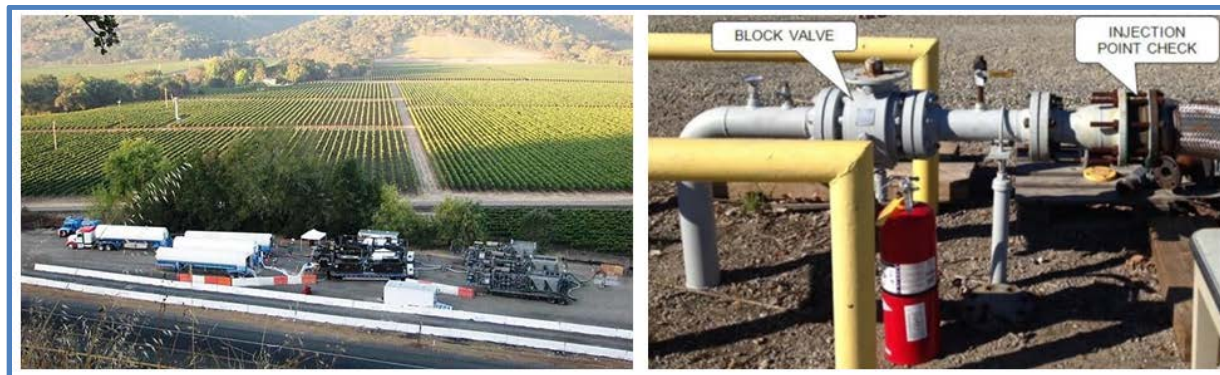
Figure 2.14 Examples of a Large-scale LNG Jobsite and an Injection Point
