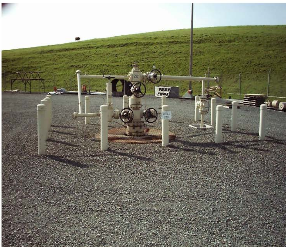
Figure N-1. A Typical PG&E Wellhead.
