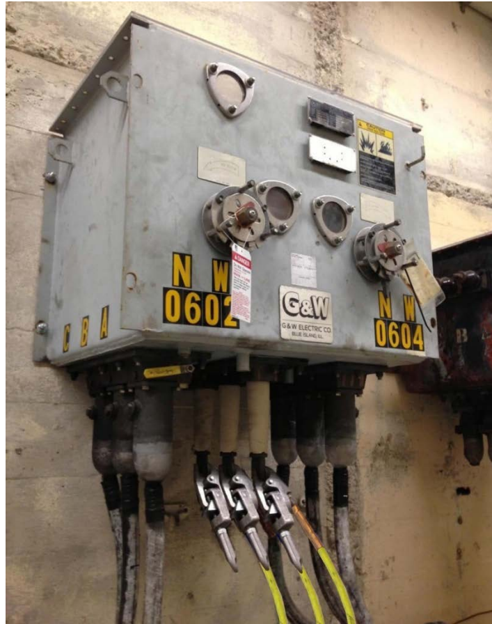
Figure C-7. TGRAM With Adjustable-Head Ground Clamps Installed on the Test-Ground Bushings.
