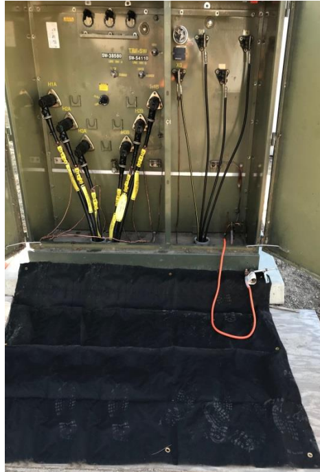
Figure 6.2. Properly Installed Ground Mat.
