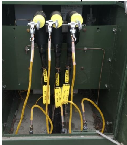
Figure 6.10. Cable Attached 2/0 Grounded Jumper
