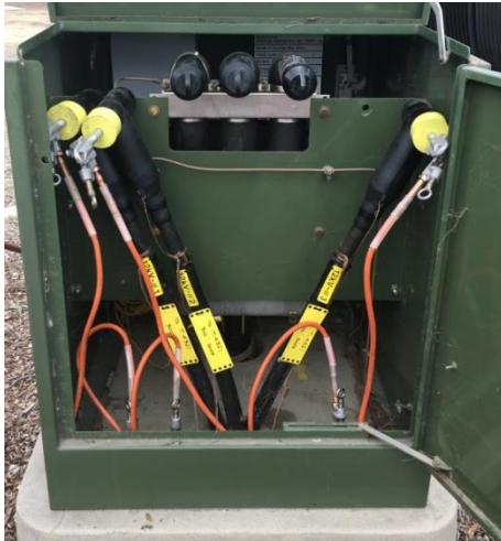
Figure 6.9. Cable Separated #2 Grounded Jumper
