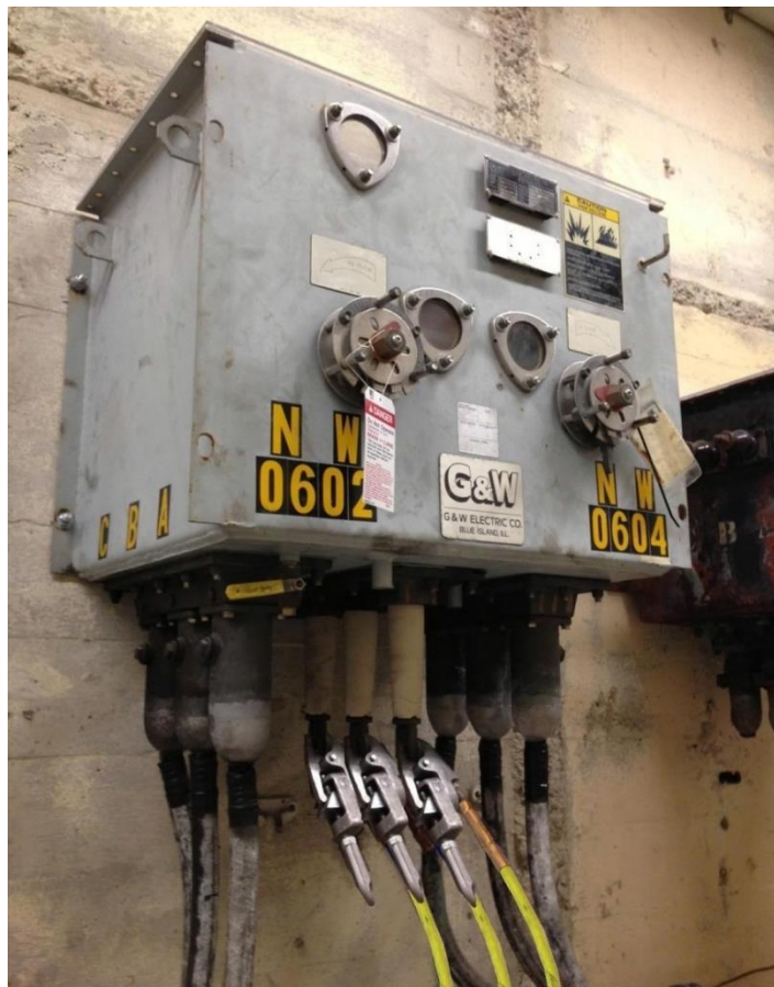
Figure 6.12. TGRAM With Adjustable-Head Ground Clamps Installed on the Test-Ground Bushings.
