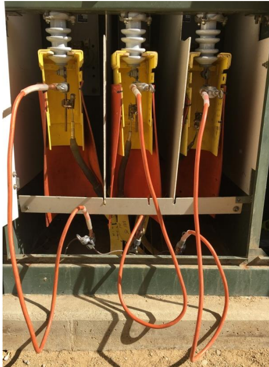
Figure 6.5. Installing Grounding Jumpers.
